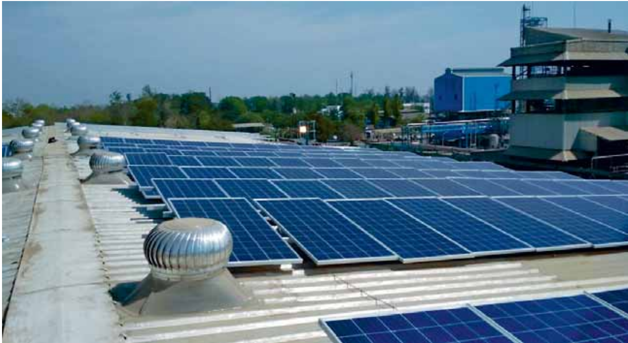
View of the solar roof top installed at Valia sulponation plant
