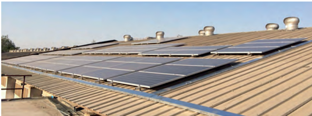
View of the Solar Roof Top Installed at Valia Factory
