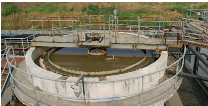
Water Treatment Plant at our Ambernath manufacturing plant
