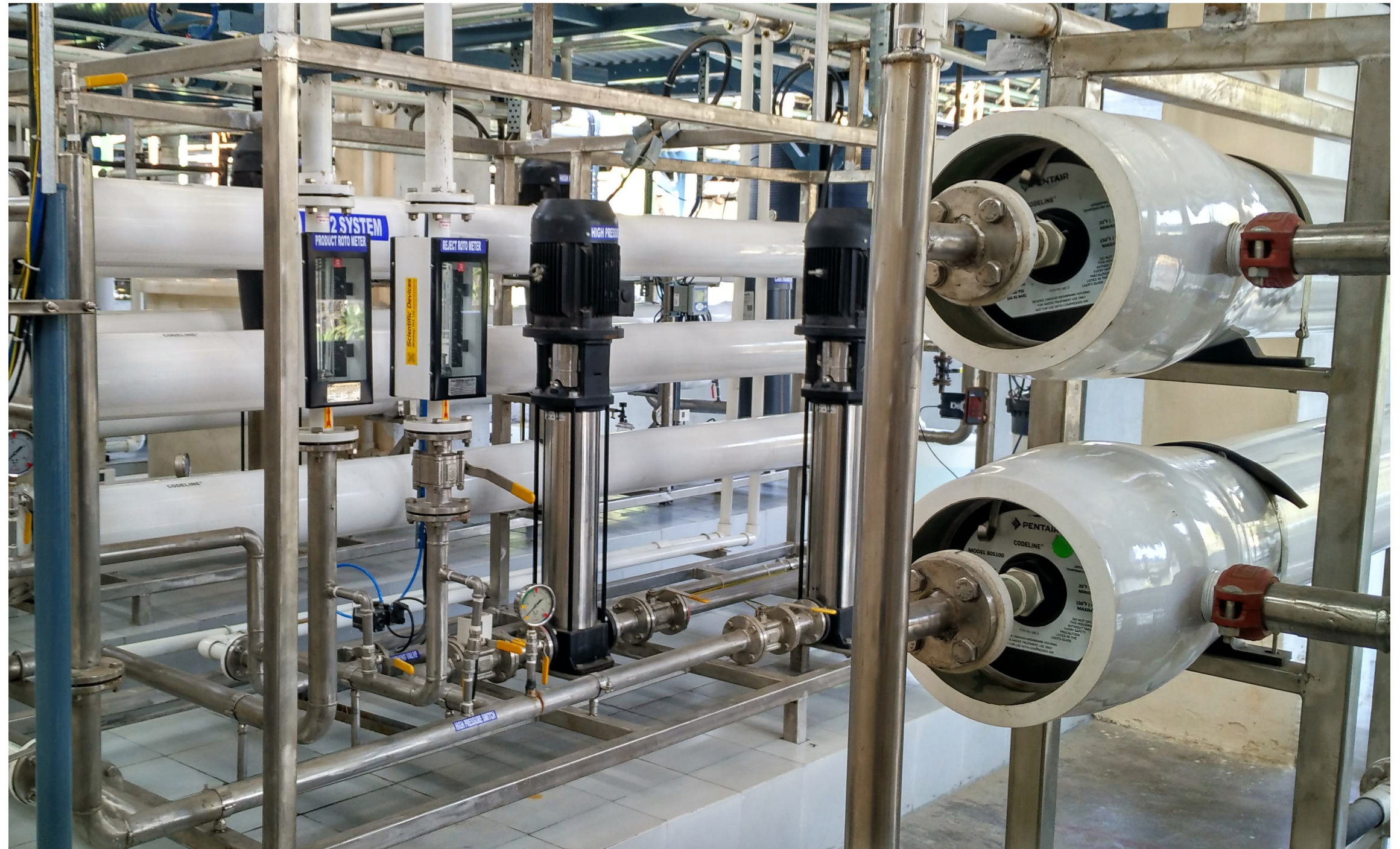
Reverse Osmosis plant at Ambernath
