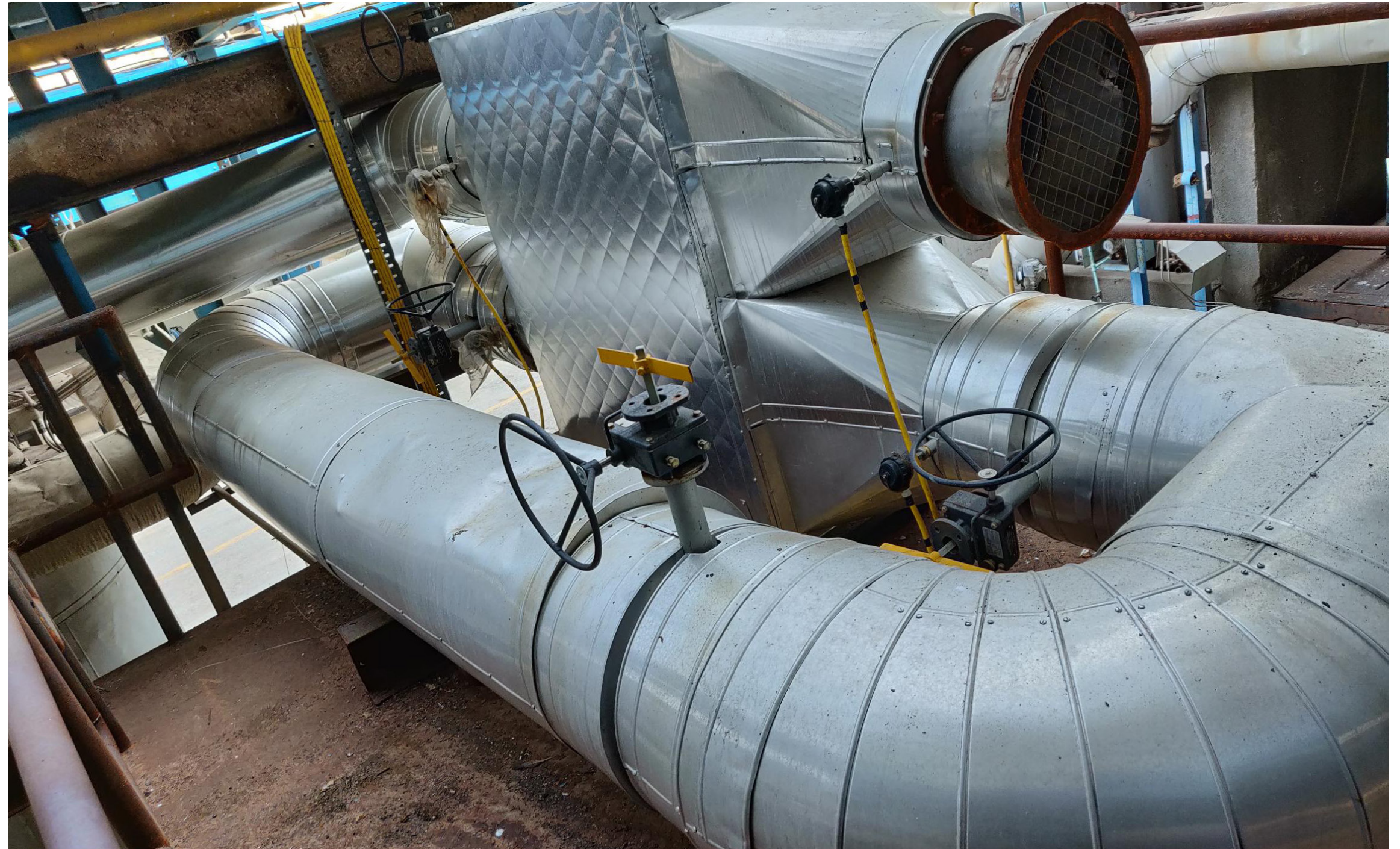
Heat pipe installed at our Valia manufacturing plant
