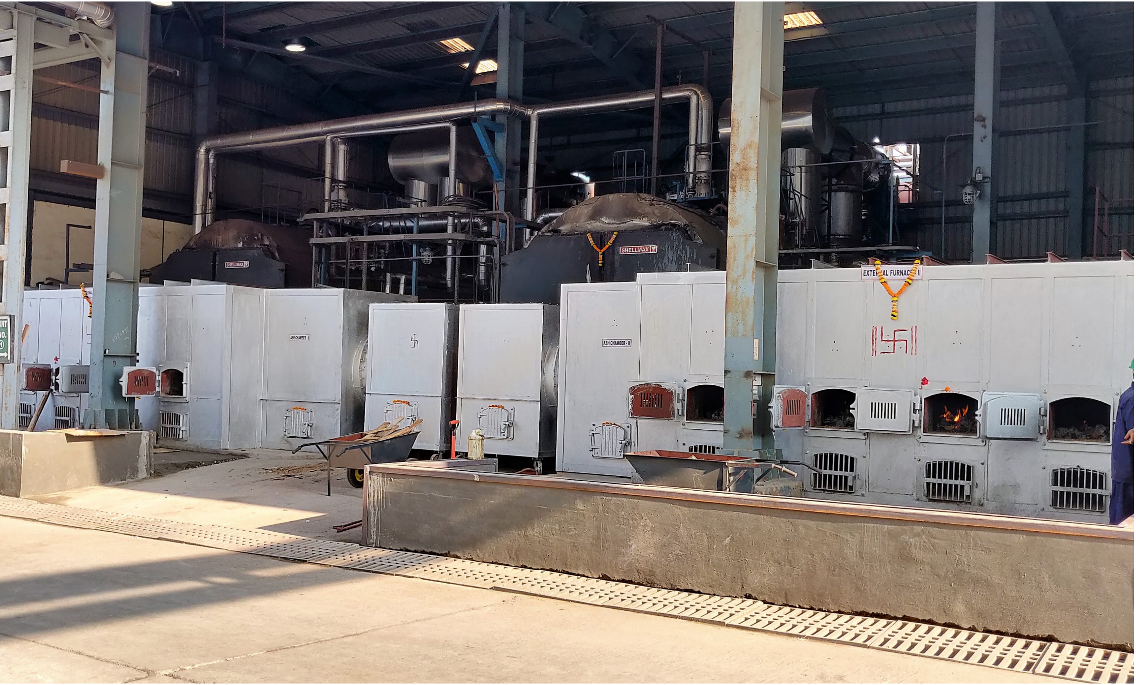
Our third briquette boiler at our Valia manufacturing plant
