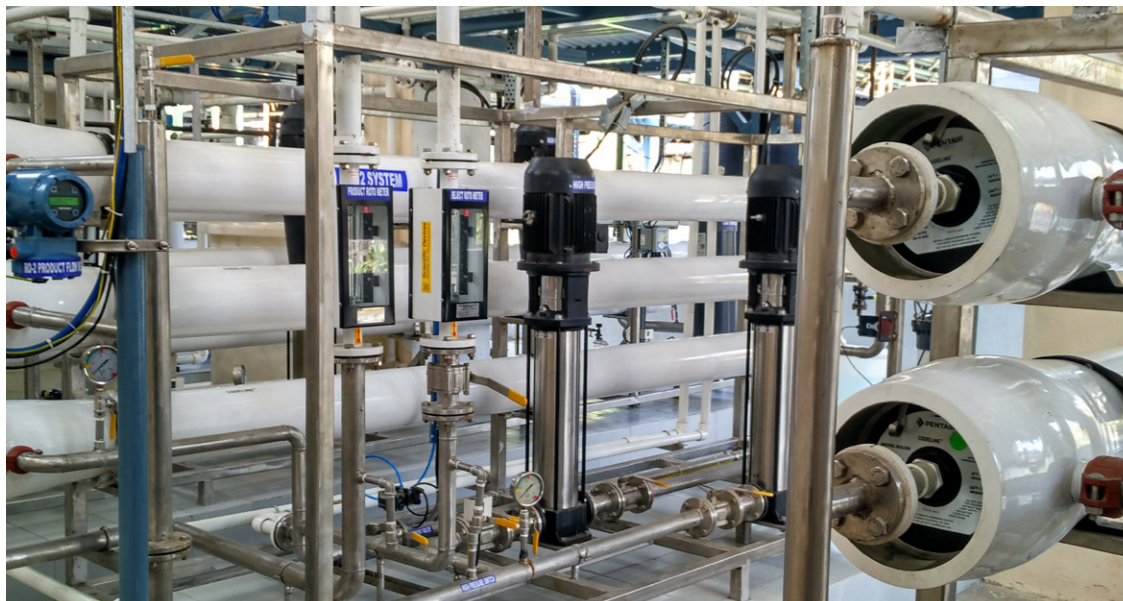
Reverse osmosis plant at Valia
