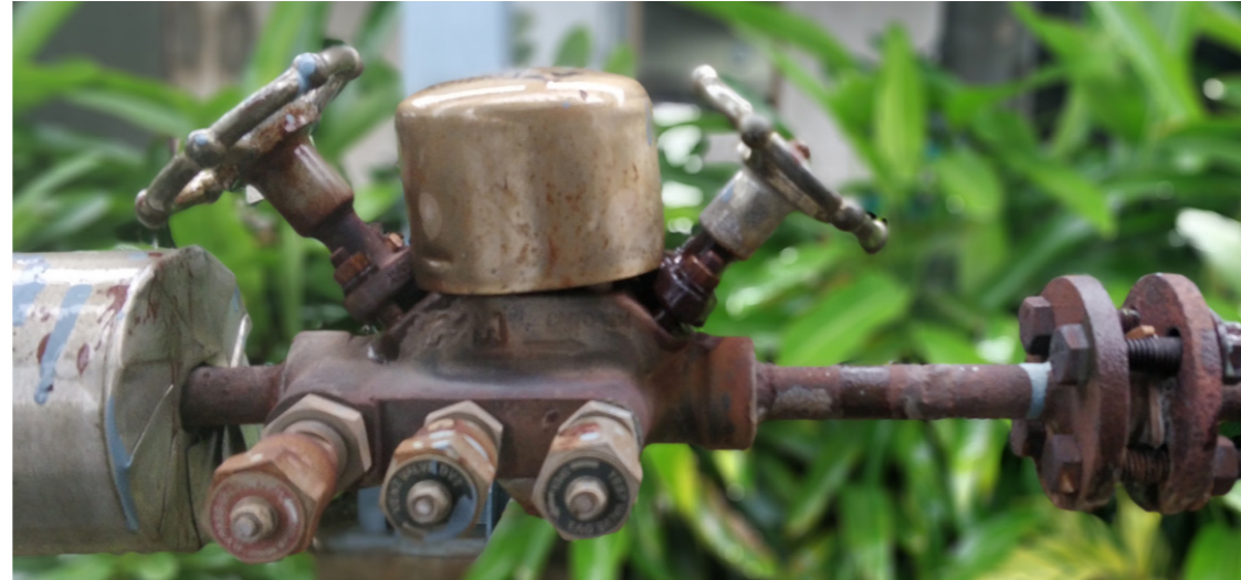
Steam trap in the condensate recovery system
