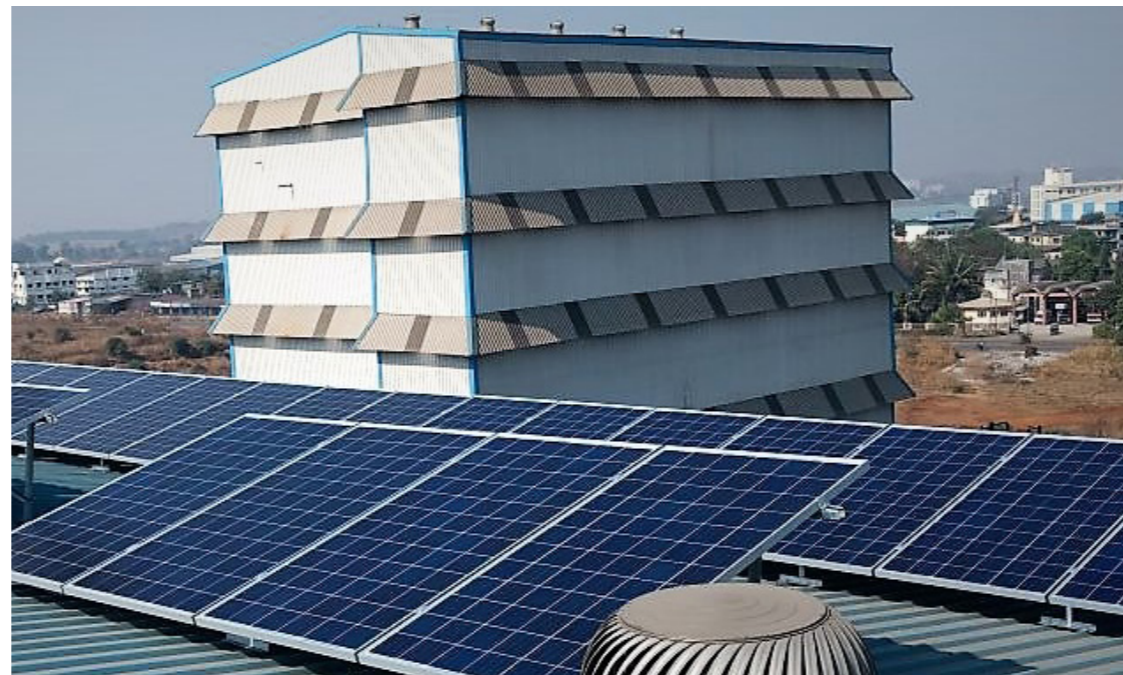
189 KW capacity solar rooftop at our Ambernath plant generates 3 lakh units of clean electricity
