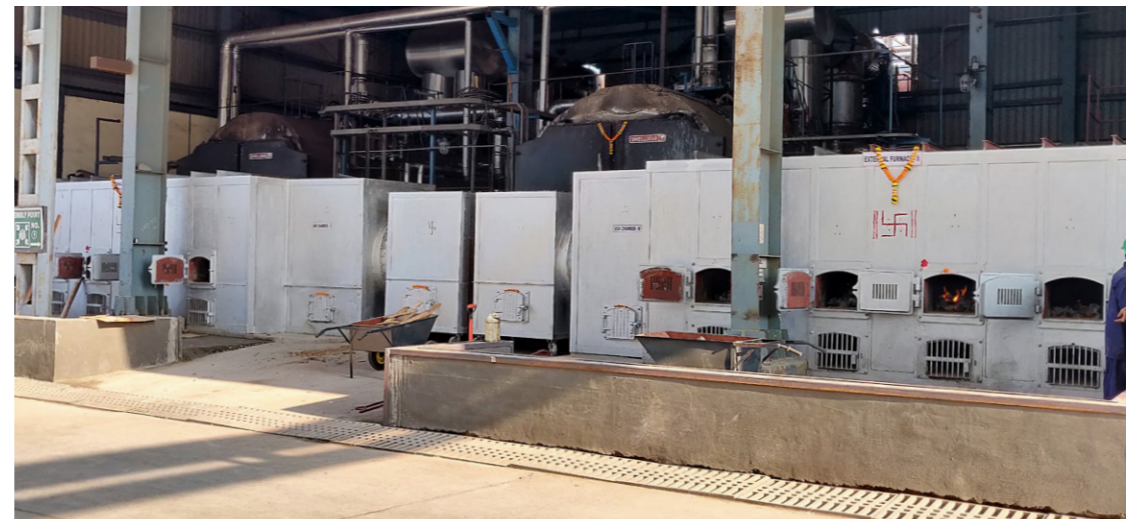
Briquette boiler at our Ambernath plant
