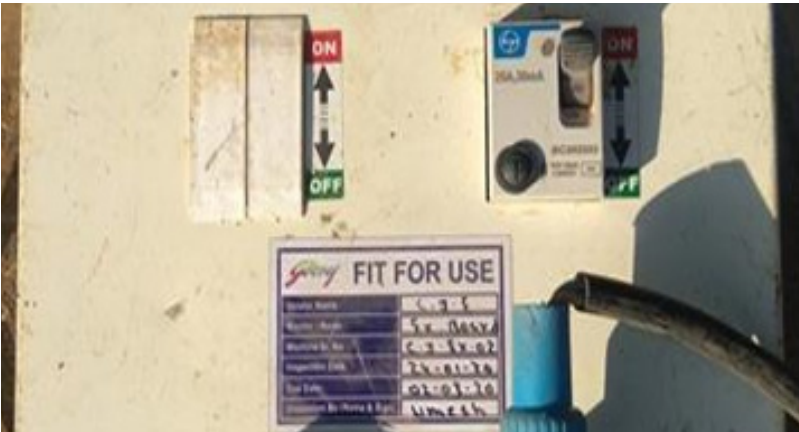
Inspection and FIT FOR USE tags on electrical boards and panels for equipment usage
